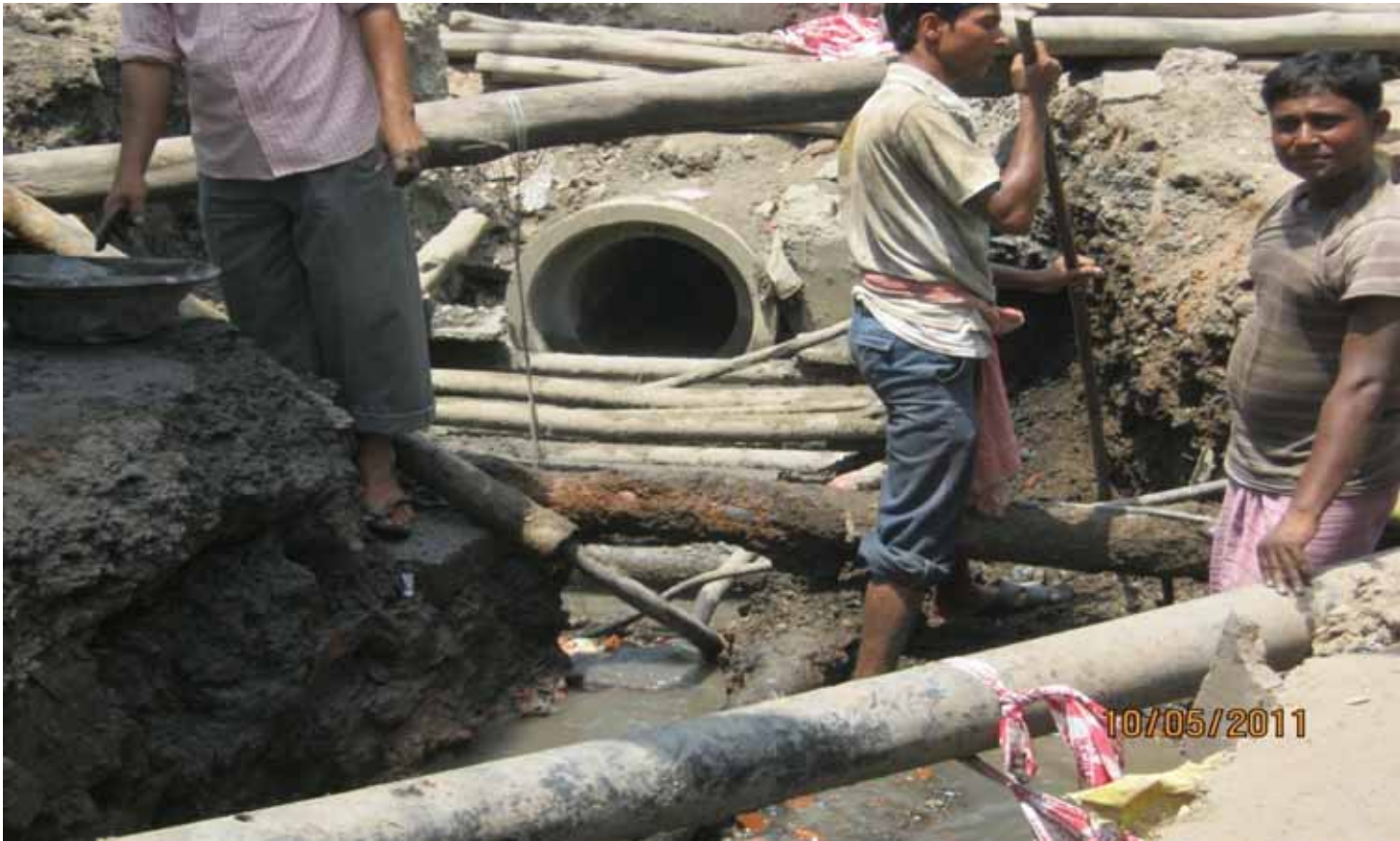
Photograph 5 Exposed Utility Services within trench at RP3
