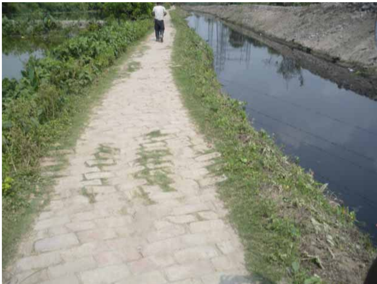
Photograph 3. Fishery Feed in EKW after re-excavation
