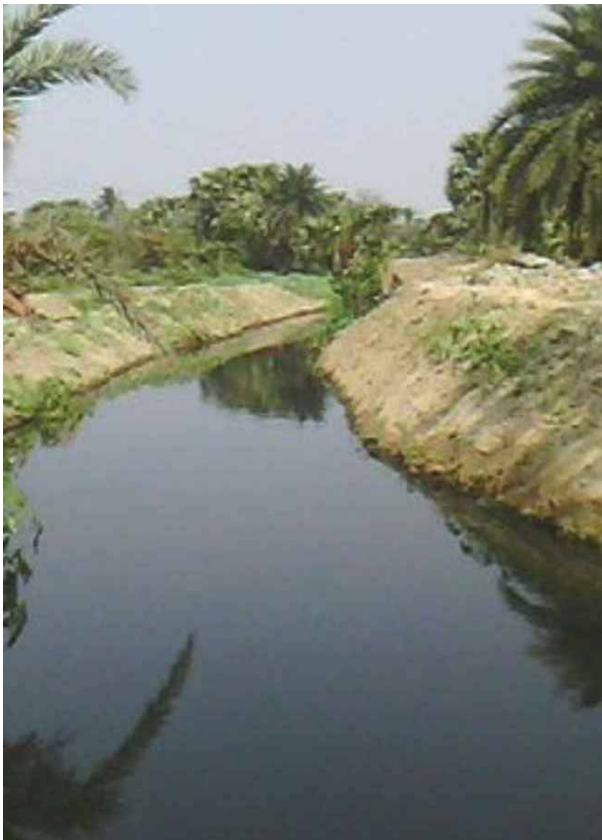
Photograph 1. Karunamoyee khal in EKW after desiltation/re-excavation
