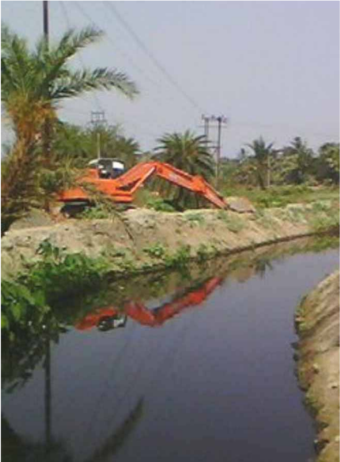
Photograph 2. Re-excavated TP- Bajbarantala khal in EKW
