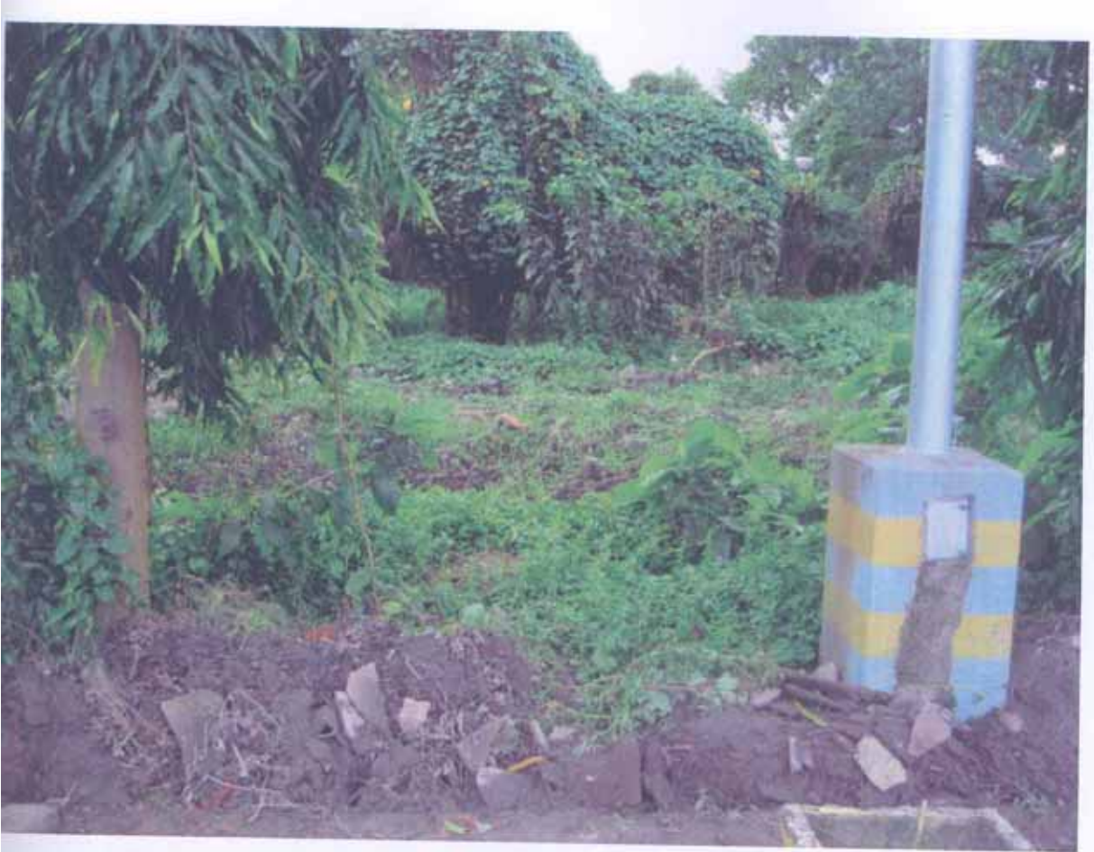
Photograph 6. Sludge Disposal Area of Garden Reach STP
